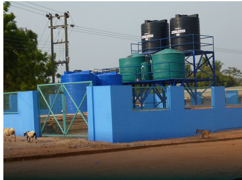
Safe Water Network's Modular Slow Sand Filtration System, Aveme, Volta Region
